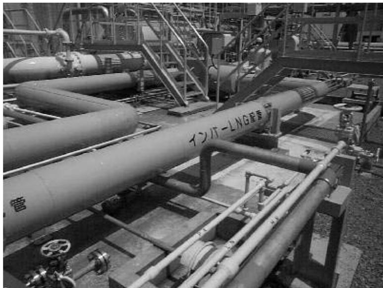
Photo 5 Invar alloy LNG piping that serves as an interconnection piping to an LNG vaporizer
