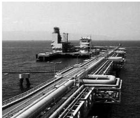
Photo. 1 Austenitic Stainless Steel Bent Piping for LNG service
