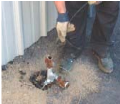
Figure 9: Installing fiber optic cable in a Toyota dealership gas service line.
