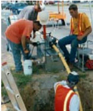
Figure 5: Direct conduit insertion using a cable jet tractor
