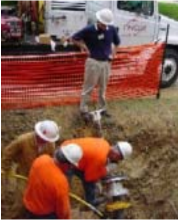
Figure 10: Installation of a 1170-foot conduit section in the Oncor-TXU pipeline.
