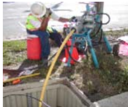
Figure 11: Fiber cable placement using standard jetting techniques.
