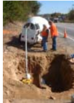
Figure 6: Conduit placement using a standard Power Rod machine
