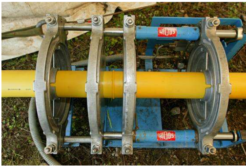
Fig. 6: Butt fusion joint
