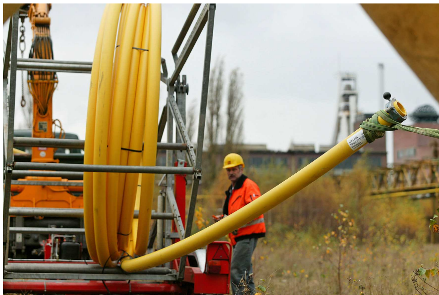
Fig. 5: VESTAMID gas pipe D110 mm, SDR-11, unrolled for test installation
