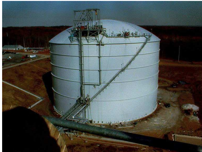
Figure 2: LNG Refrigerated Storage Tank
