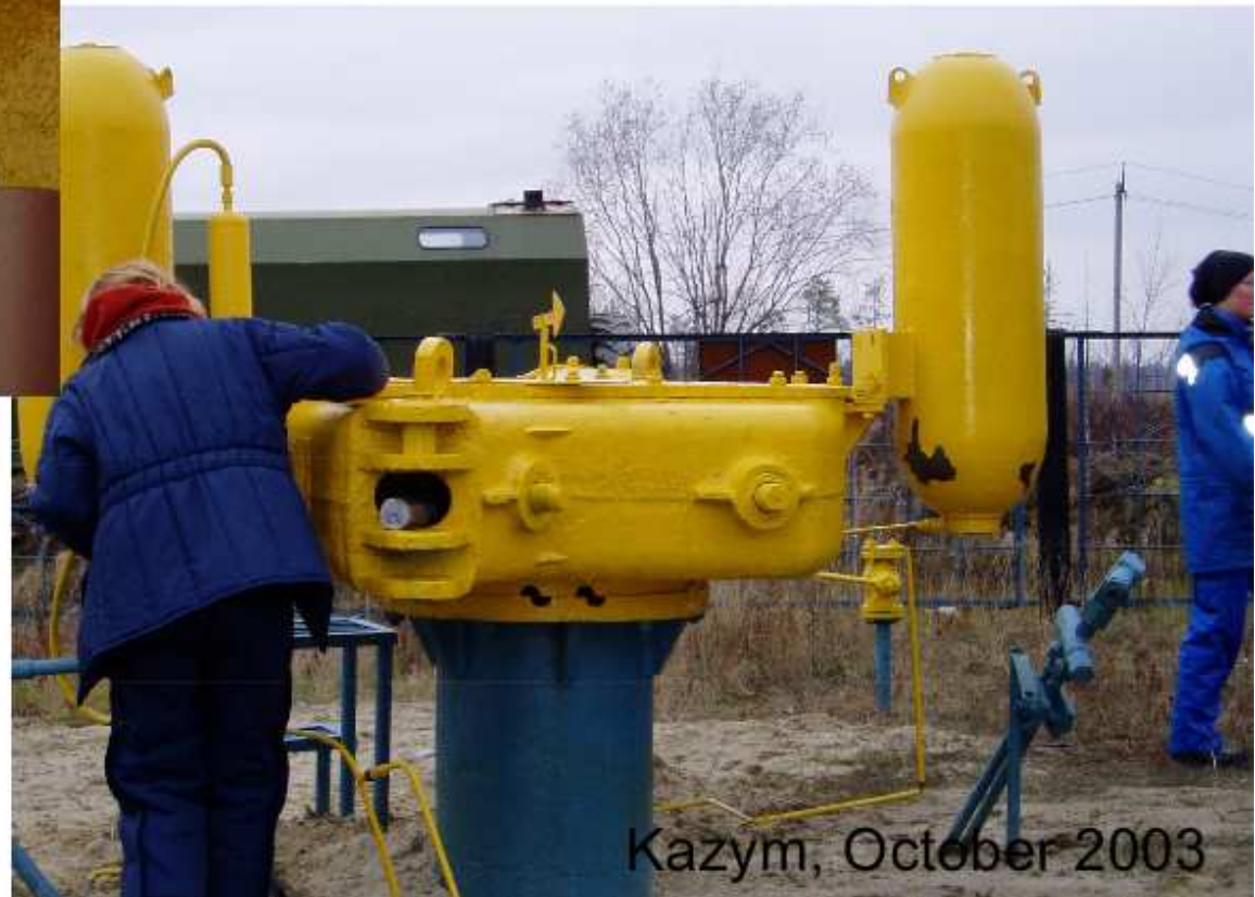
Screening at pipeline intersection
