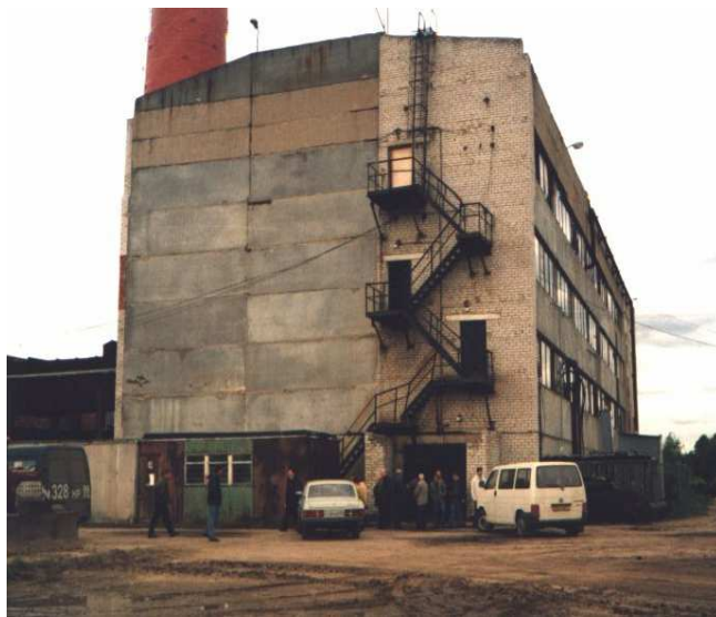
Central Heating Station Kaljasin
