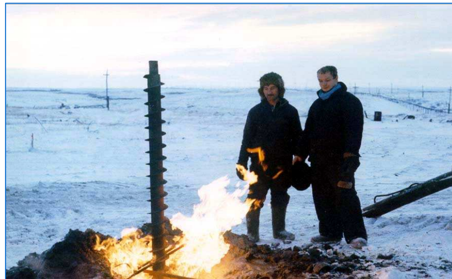
Gas fire from permafrost hydrates when drilling monitoring well
