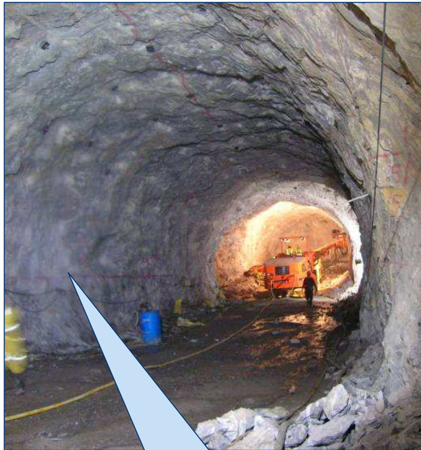
Shotcrete coating used to minimize risk of falling rock
