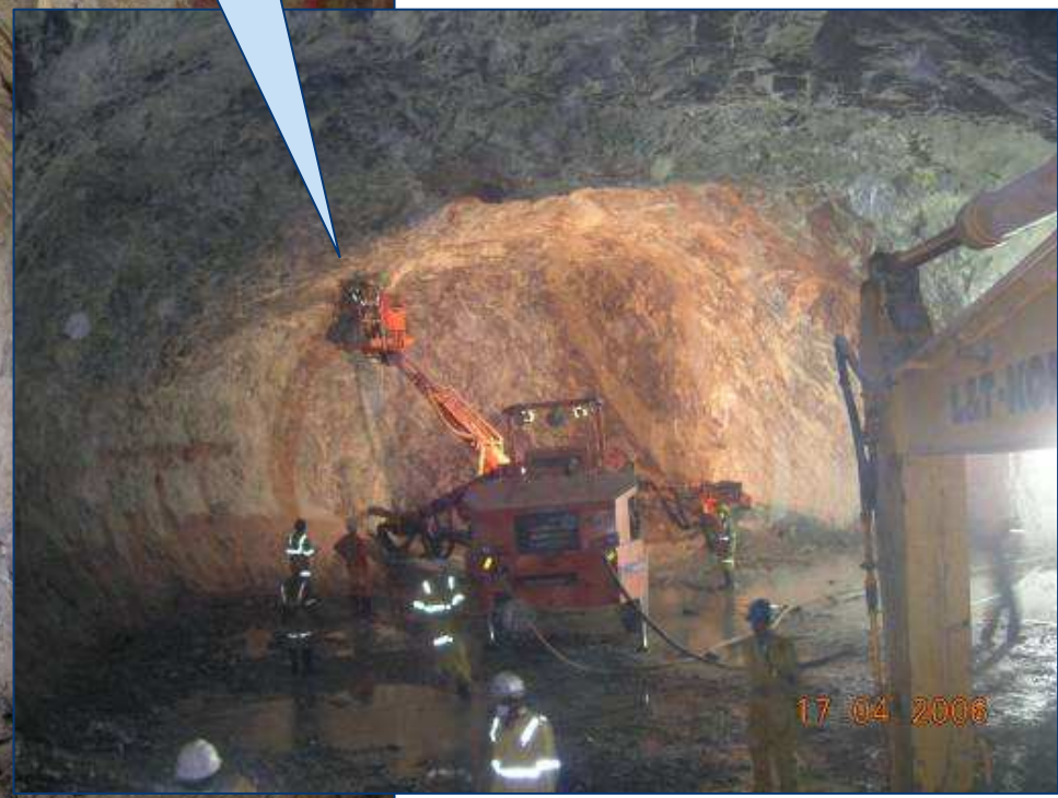
Shotcrete coating used to minimize risk of falling rock
