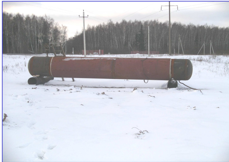
Pipe with installed repair construction is ready for testing
