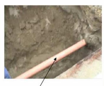
Replace Section of 4" Aldyl-A Pipe for 4"x2" Branch Saddle Installation
