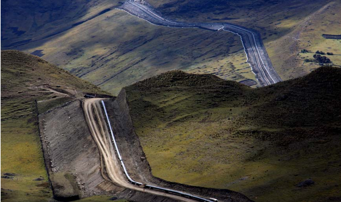
PERU LNG pipeline string ready for lower-in (June 2009)
