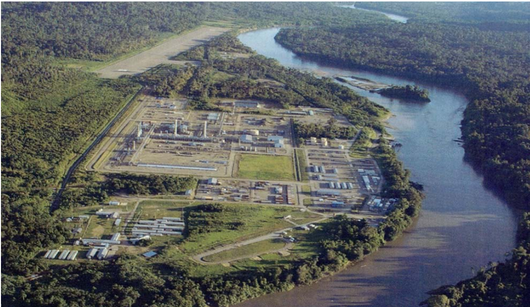
Malvinas gas production Plant in the Amazon jungle
