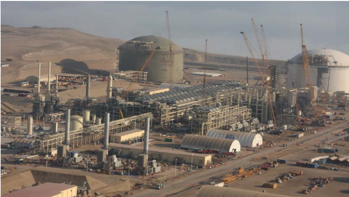
Liquefaction Plant overview (June 2009)
