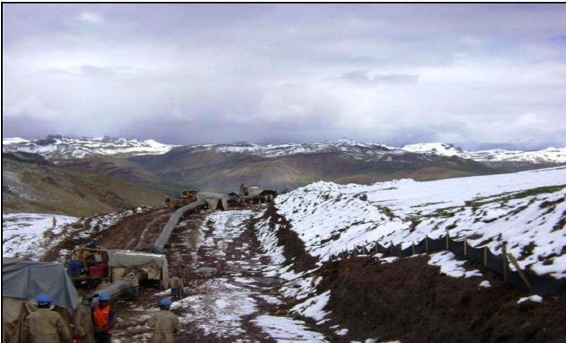
Pipeline construction during summer 2009 at the Andes
