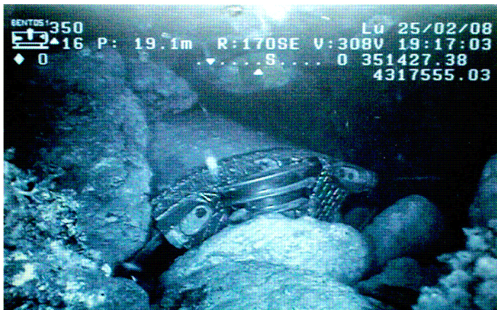
Figure 8.04 Ibiza Landfall Tunneling Exit Point
