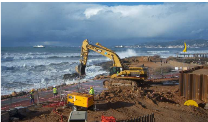
Figure 8.07 Mallorca Landfall Onshore Excavation
