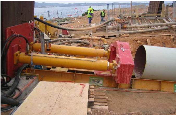
Figure 8.02 Ibiza Landfall Tunneling Machine
