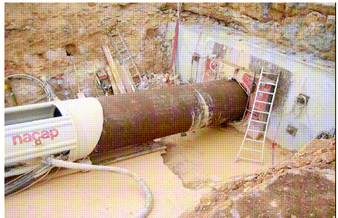
Figure 8.03 Ibiza Landfall Tunneling Operations
