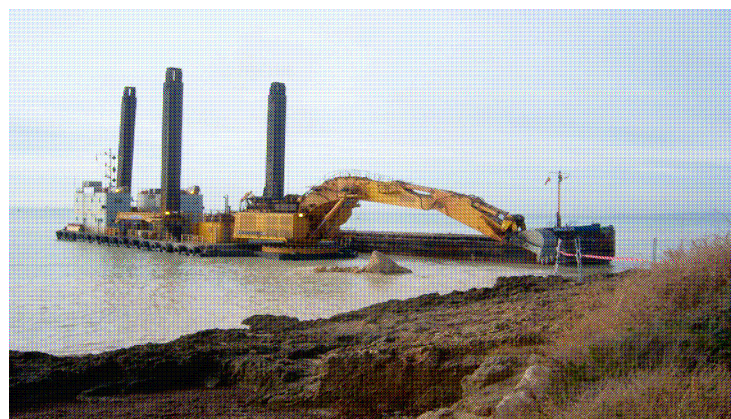
Figure 8.08 Mallorca Landfall Nearshore Dredging
