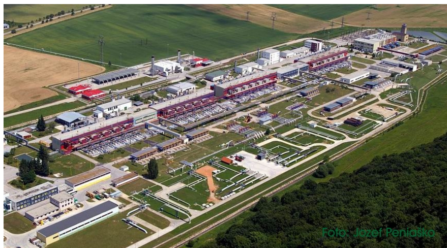
Figure 2. Compressor station 02, Jablonov nad Turňou
