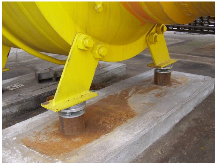
Figure 12. Vibro-insulation supporting structures under foot of ball-valve
