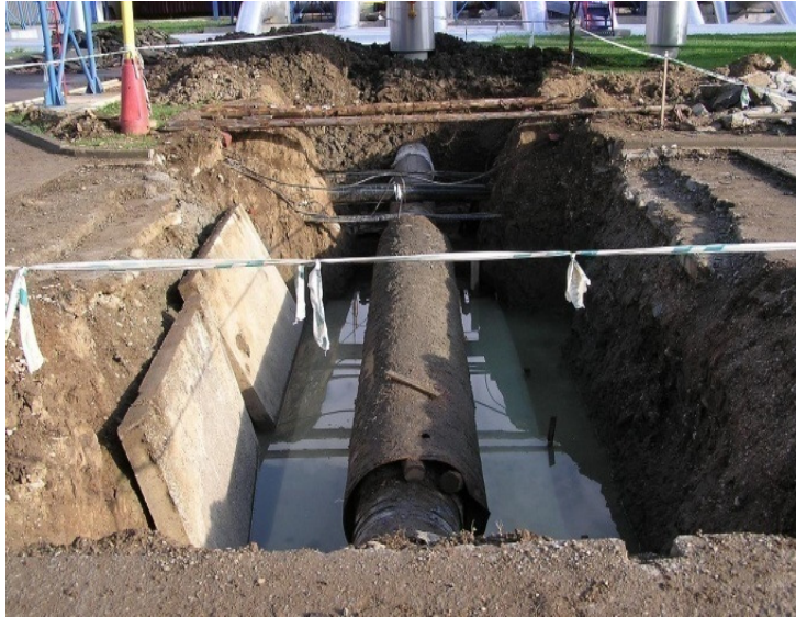
Figure 11. Casing condition after excavation
