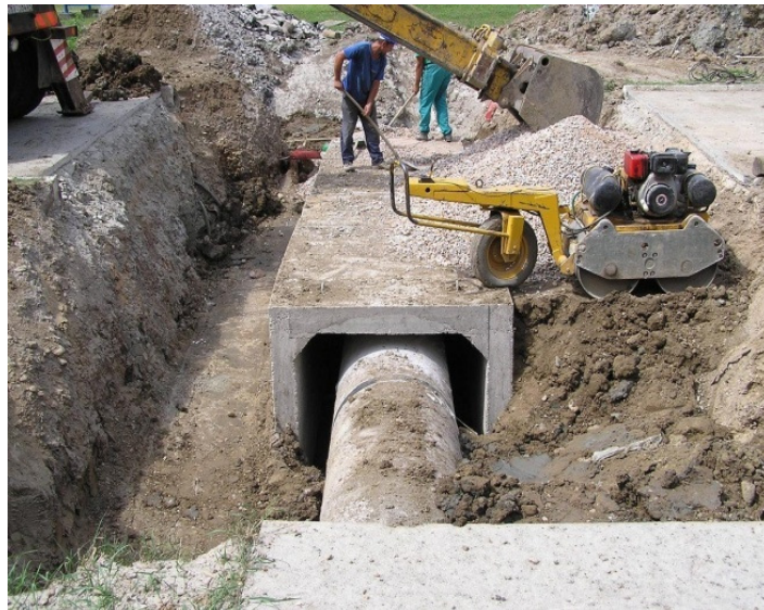
Figure 12. Repair of casing by replacing it with concrete prefabricate
