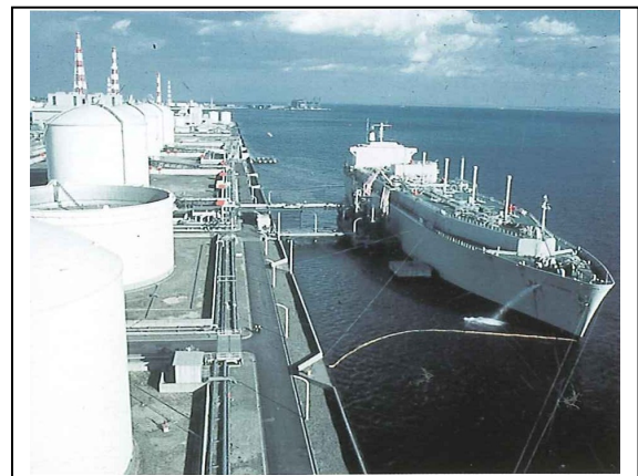
Fig. 2-2 First acceptance of LNG in Japan (Negishi terminal of Tokyo Gas (November, 1969))
