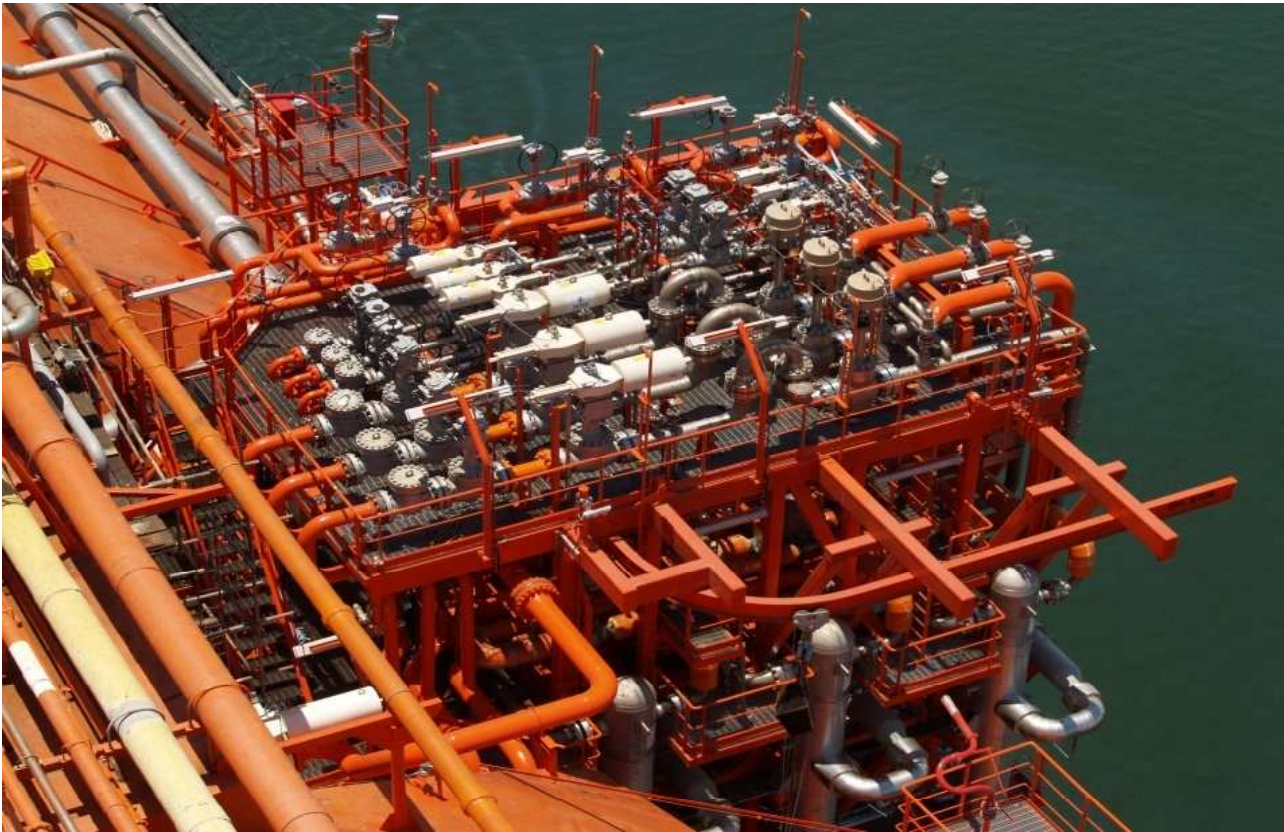
Figure 6 – The regasification unit aboard the Golar Spirit
