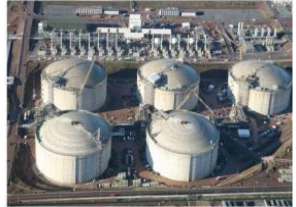
Storage Tanks at South Hook Terminal
