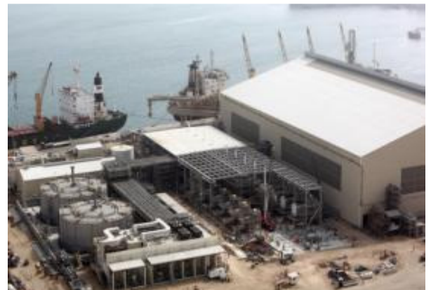
Common Sulfur Storage Facilities
