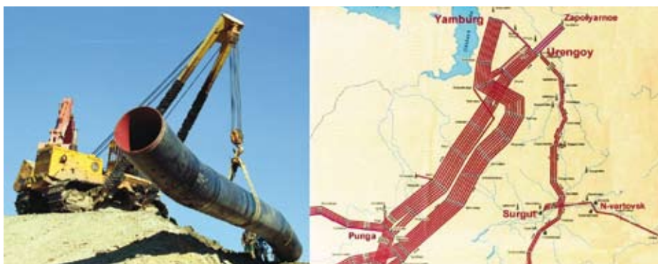
Fig. 3.11: From the laying of the Gazprom Bluestream pipeline (left). The pipeline is buried in a deep trench and leaves only a limited visual footprint once buried. The map to the right shows the incredible concentration of large diameter (56"; 1,40 meter diameter) pipelines in the Urengoy and Yamburg areas of northern Russia. This is part of the huge infrastructure of gas pipelines around the world. (Source: Gazprom).
