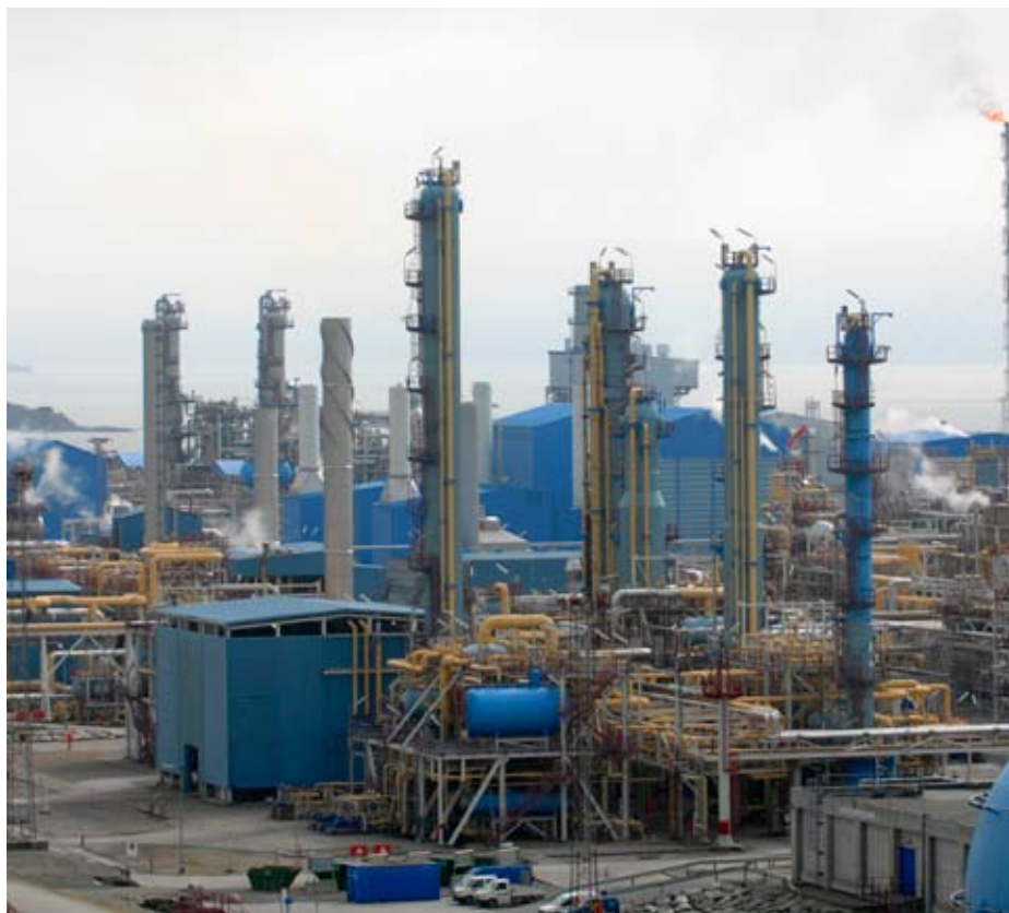
Fig. 5.1: Natural gas processing plant with gas/liquids separation columns, compressors, storage tanks etc. at Kårstø, Norway (Picture: Øivind Hagen/StatoilHydro).
