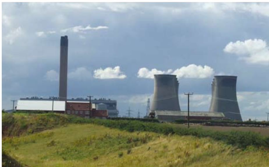
Fig. 4.6: Coal fired power plants generates 72% of all power generation CO 2 . Here the Eggborough power station in UK. Modernising the power sector by replacing aging coal fired power plants by state of
