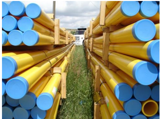
Figure 4 – 4" PA12 pipe supplied in both coiled and 50' long sticks
