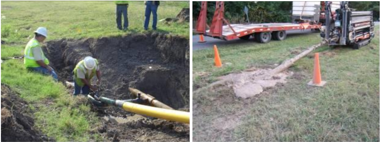
Figure 10 – Using directional drilling to install the PA12 under a roadway
