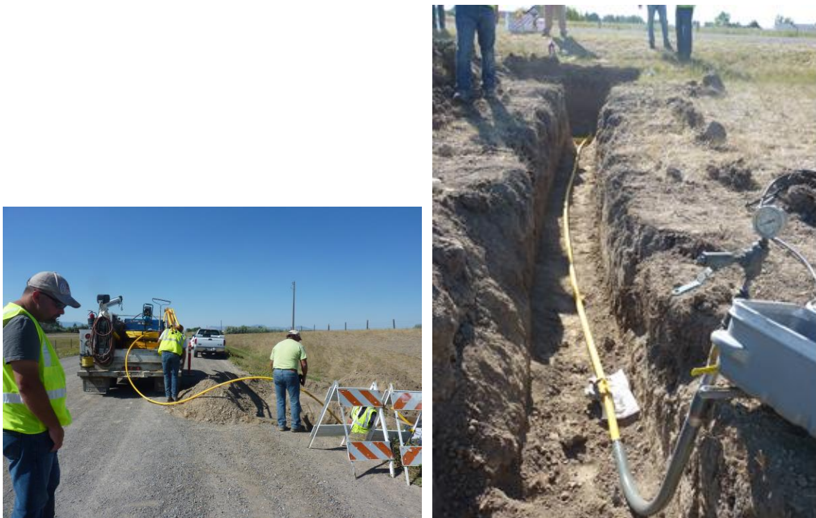
Figure 8 – Installing the PA12 services
