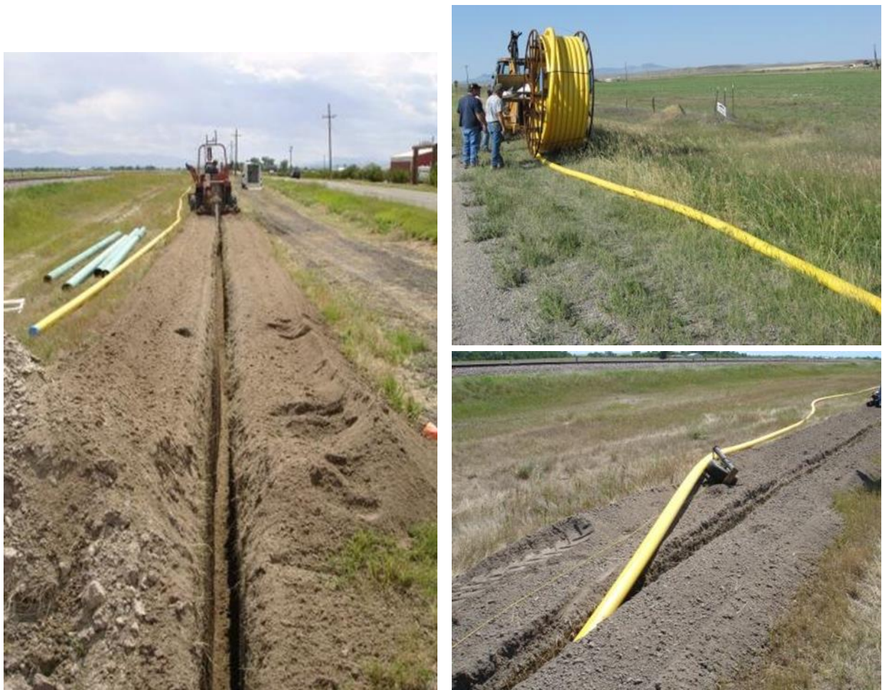
Figure 6 – Installing the 4" – PA12 Piping system in Montana (Energy West)
