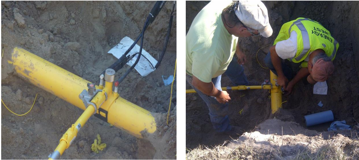
Figure 7 – Installation of PA12 electrofusion service tees and other service components
