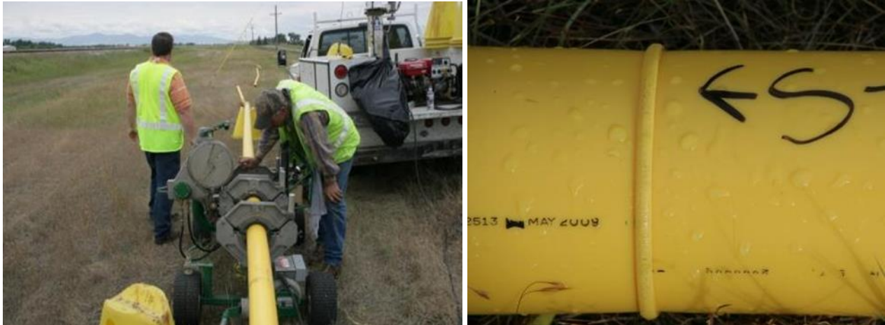
Figure 5 – PA12 was butt fused using traditional equipment and methods
