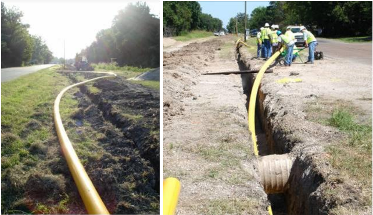
Figure 9 – Installation of the 6-inch PA12 pipe in Greenville, MS
