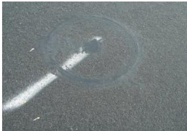
Figure 2. Keyhole pavement restoration
