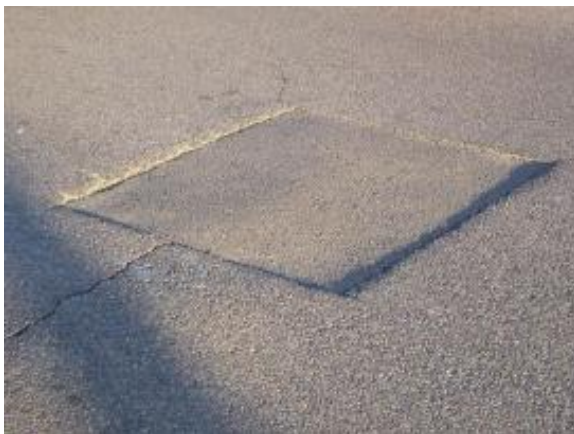
Figure 1. Traditional utility restoration
