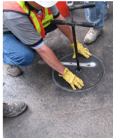
Figure 5. Pavement core being reinstated after the underground work has been completed,
