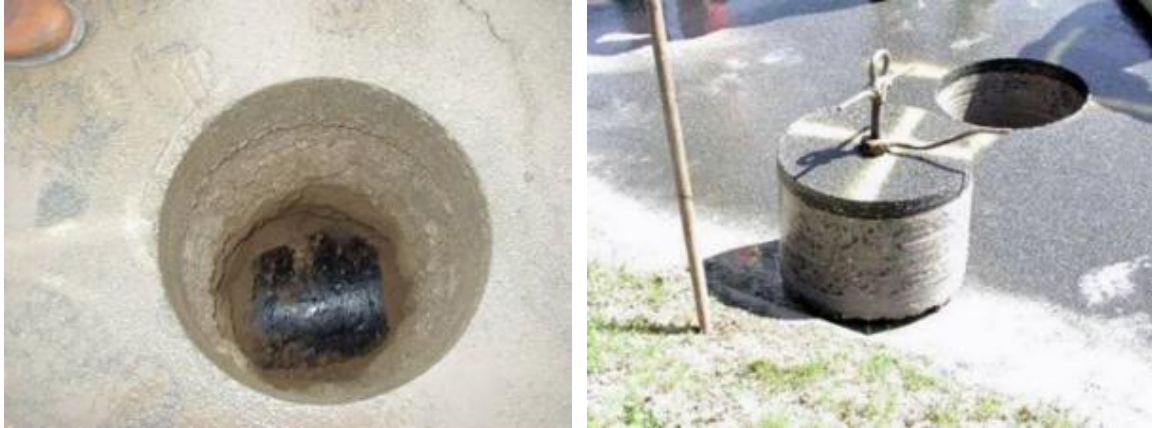
Figures 3 and 4. Pavement coring to expose underground utilities
