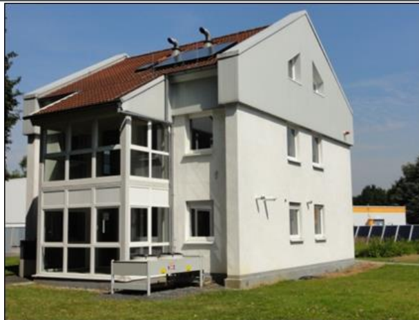
Figure 1: External View from GWI's test house [3].
