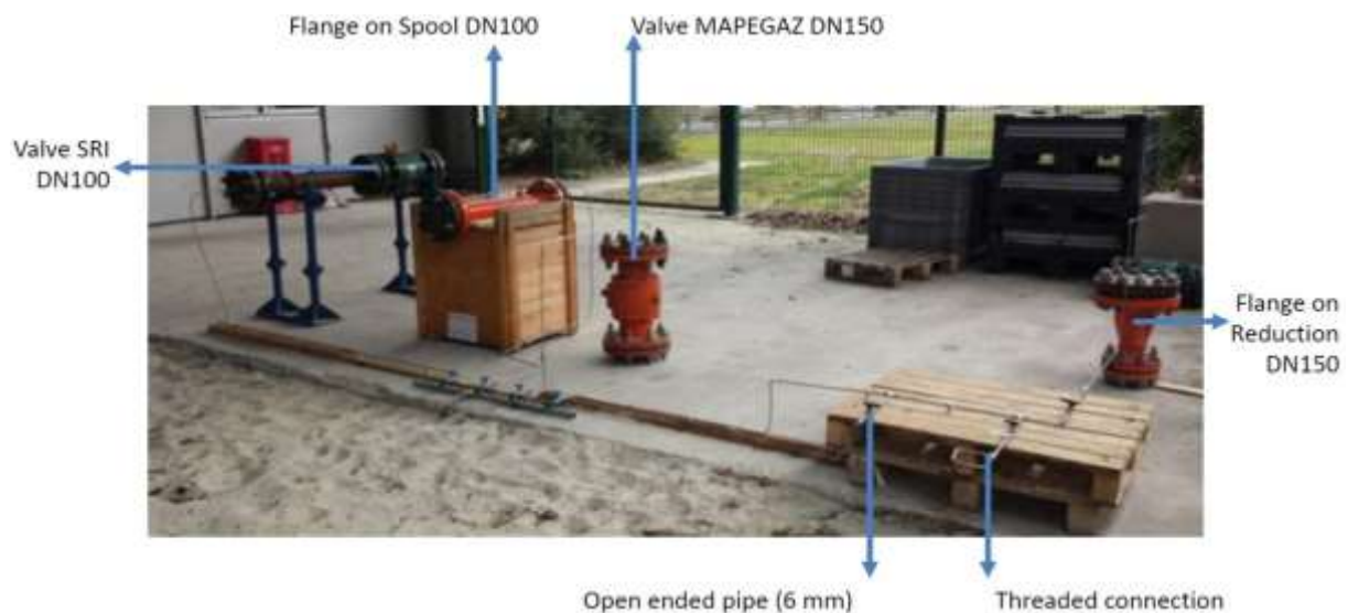
Fig.2 Picture of the second part of the test facility
