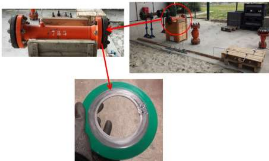
Fig.3 Creation of a leakage - damaged metallic gasket and graphite packing, two bolts bad fitted on the same flange
