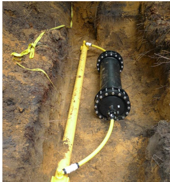
Figure 11 – Test rig under G-gas conditions.
