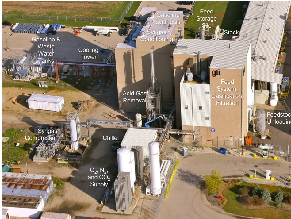
Figure 1. GTI's Flexible, Feed-to-Product Platform for Integrated Pilot-scale Demonstration of Energy Conversion Technologies
