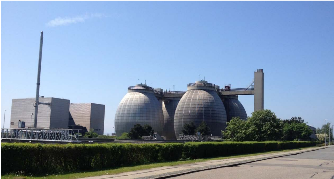
Figure 2. Biofos Waste-Water Treatment Plant Located in Copenhagen, DK (the anaerobic digester units are located in the center of the photo)
