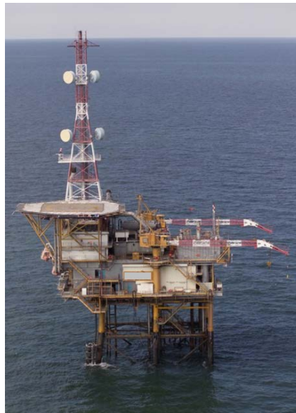
Figure 9 – Main Process/Compression Platform for Gas Cluster
