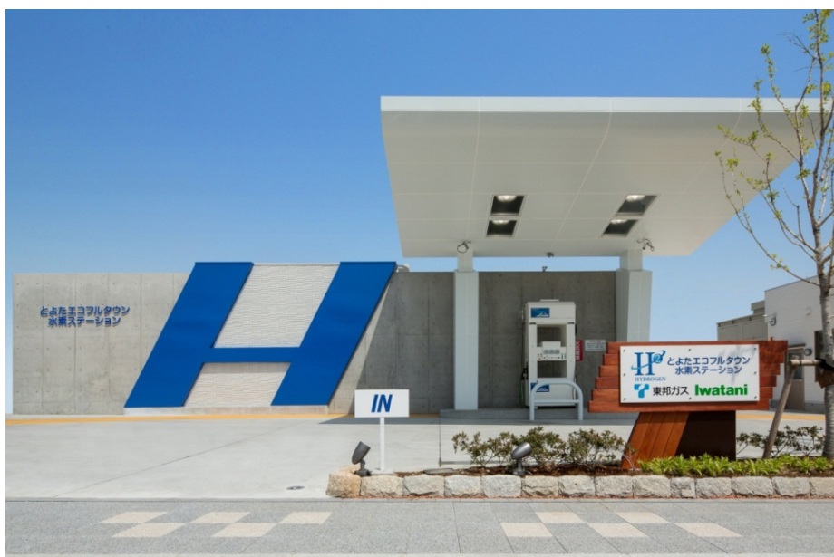
Figure 4. Outside Appearance of Toyota Ecoful Town Hydrogen Refueling Station
