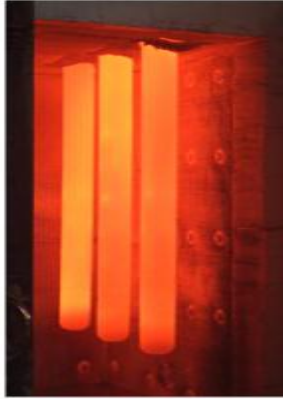
Figure 3: Single-ended RT Burner Installations within Furnace
