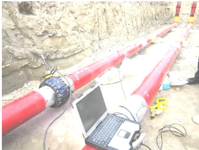
Figure 5. Installation of piezoelectric type sensor
