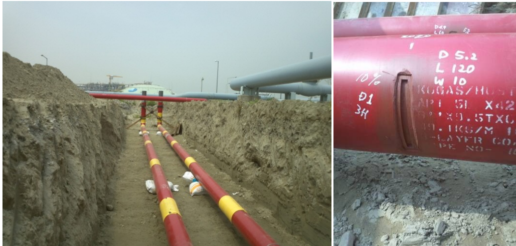
Figure 1. Test pipe installation and artificial defects
