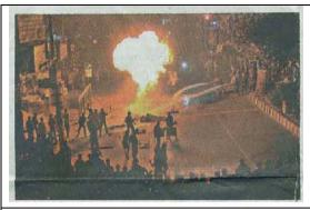
Gas Line punctured and caught fire during laying of a internet cable line underground at farm Gate intersection of the City of Dhaka
