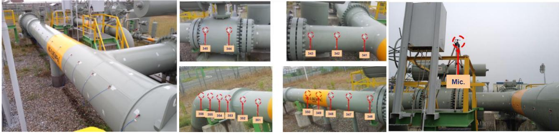
Fig. 2 Measuring point for vibration and sound pressure
