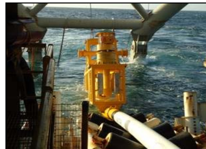
Figure 15. Exit of the ILS throughout the stinger
