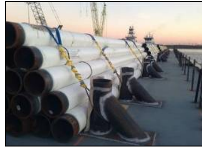
Figure 2. 16” gathering pipeline
