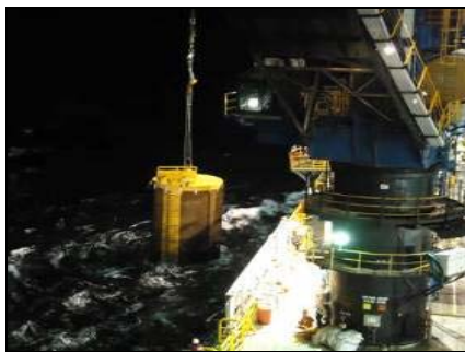
Figure 10. Lowering of the suction pile
