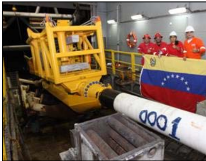
Figure 11. PLET 1 installation welded to the first joint
