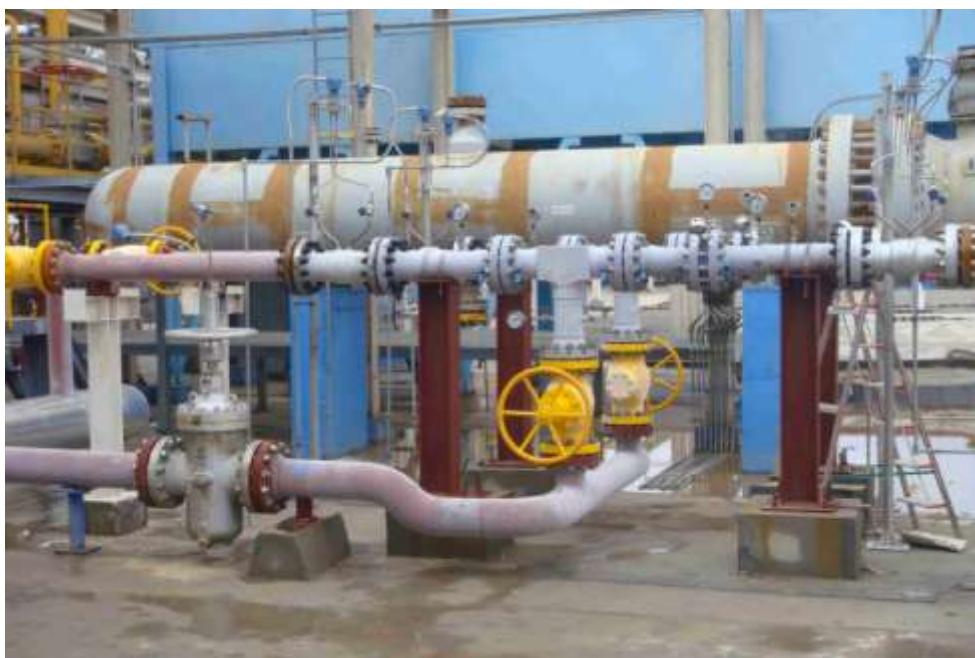
Fig.3 3S-separation unit at YAHA field («Petrochina»)
