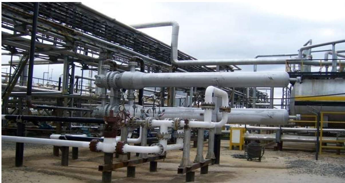
Fig.2 3S-separator at Gubkinskoe CGTP, JSC "Rosneft"
