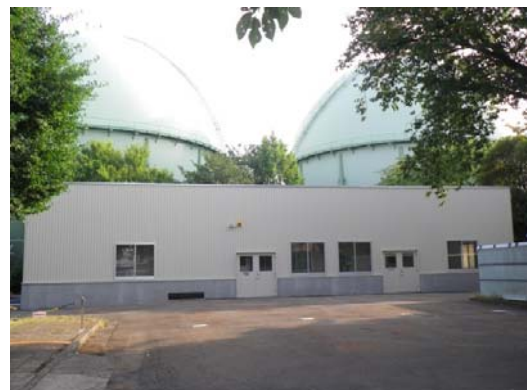
Photo 7 Governor station after reinforcement work
