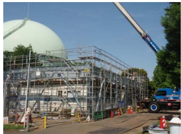
Photo 9 At upper frame (steel) construction work
