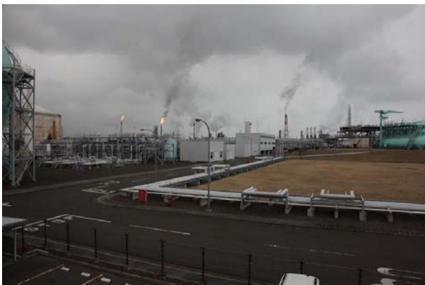
Photo 3.1 LNG terminal before the strike of the tsunami of the Great East Japan Earthquake in 2011.
