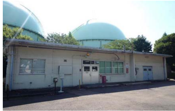
Photo 6 Governor station before reinforcement work
