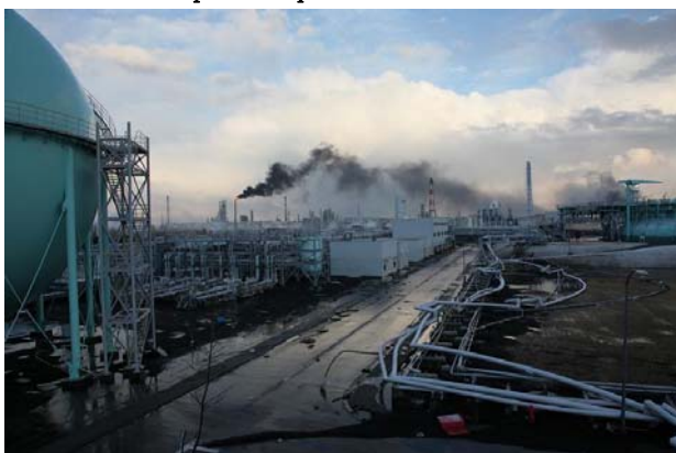
Photo 3.3 LNG terminal after the strike of the tsunami of the Great East Japan Earthquake in 2011.
