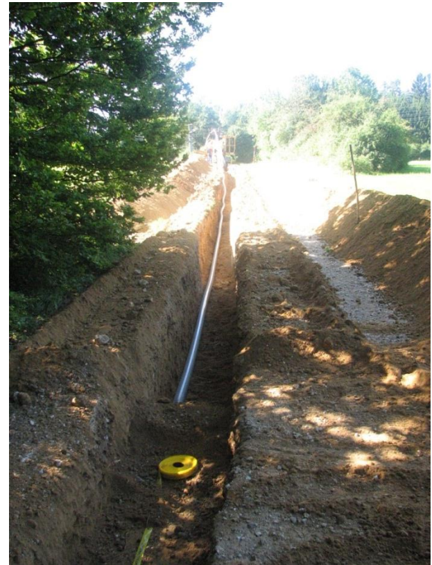
Pipe trench with HexelOne® pipeline and warning tape
