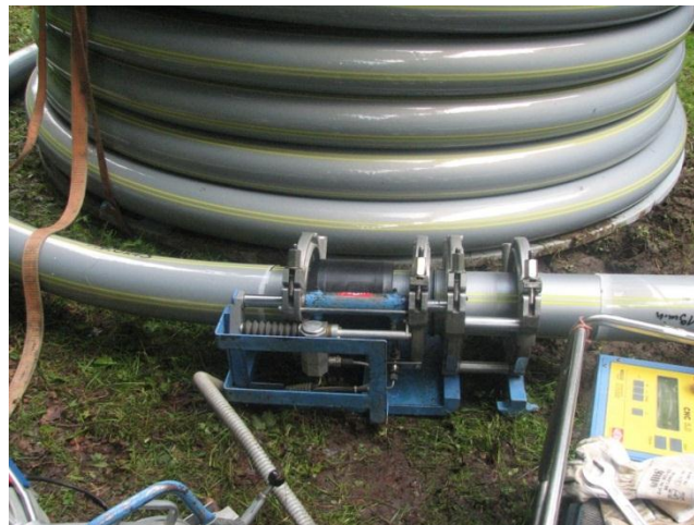
Fusion welding in the field
