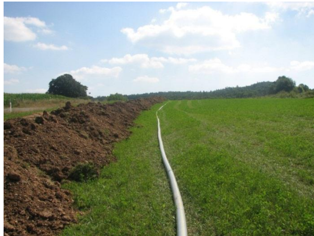
Pipeline laid out prior to installation
