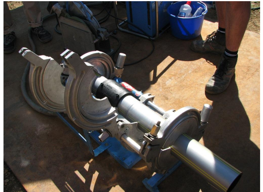
Welding with automatic welder
