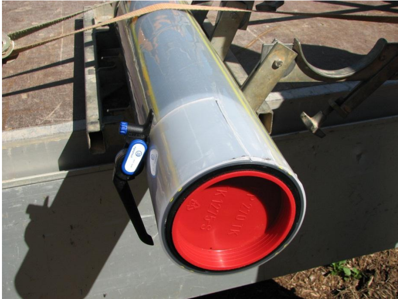
Removal of protective sleeve prior to welding
