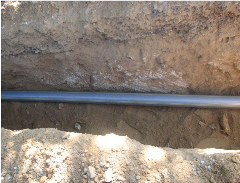
Installation in category 7 soil
