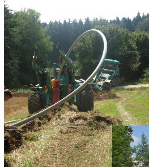
Installation by ploughing
