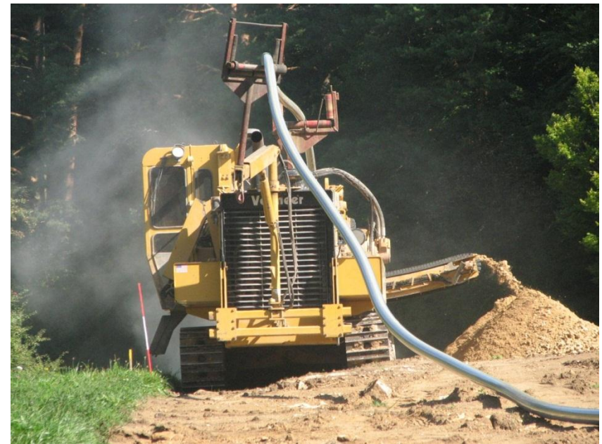
Cutting of trench with simultaneous installation of pipe
