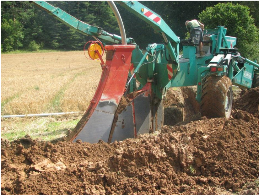
Installation of plastic pipe incl. warning tape by ploughing
