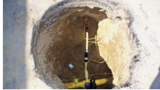
Connect 1/2" tube to service tee
