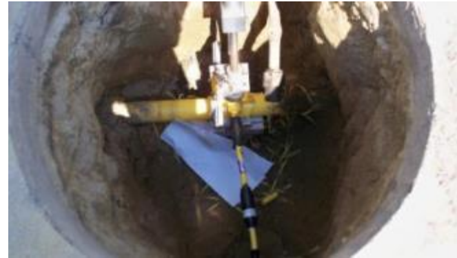
Completed service transfer
