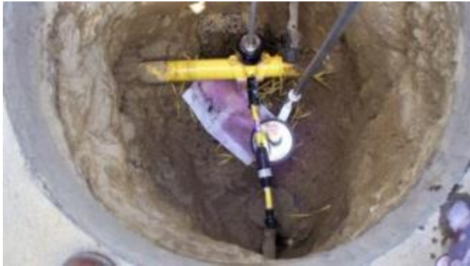
Soap test new service connections
