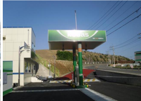
Guangyang LCNG Station
