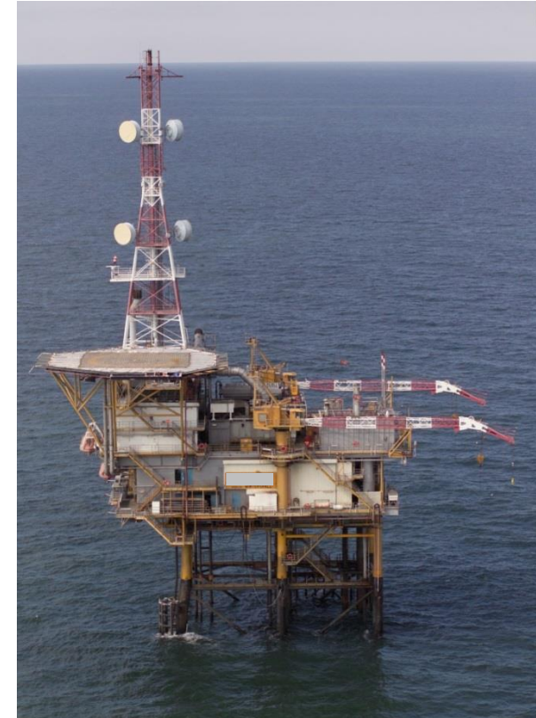
Process/Compression Platform Now Satellite
