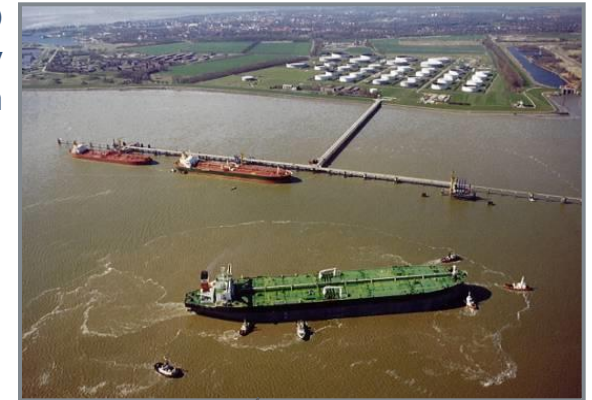
NWO crude oil jetty and tank farm
