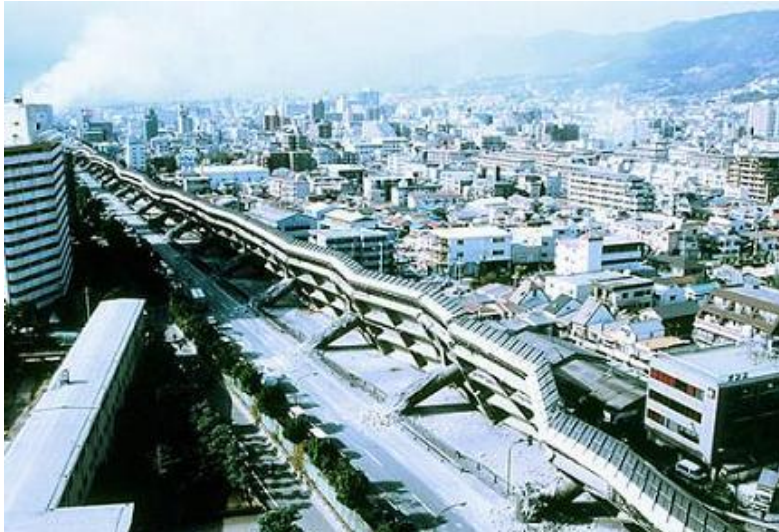
The Southern Hyogo Prefecture Earthquake (1995)
