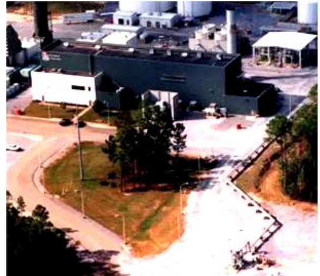
Alabama Electric Cooperative's CAES Plant (110 MW-26 Hr) Plant Commissioned: June 1, 1991 Air Store: Solution Mined Salt Cavern
