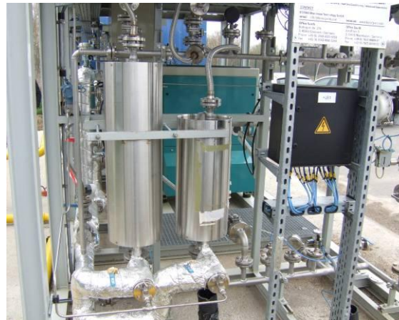
Skid-Mounted Gas Separation Unit 8 m x 3 m x 3,2 m (L x W x H)
