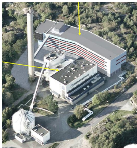
GoBiGas phase 1 20 MW SNG Demonstration plant Gothenburg Energy/E.ON
