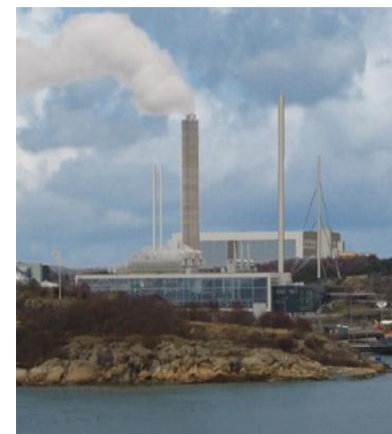
GoBiGas phase 2 80 MW SNG Commercial plant Gothenburg Energy/E.ON
