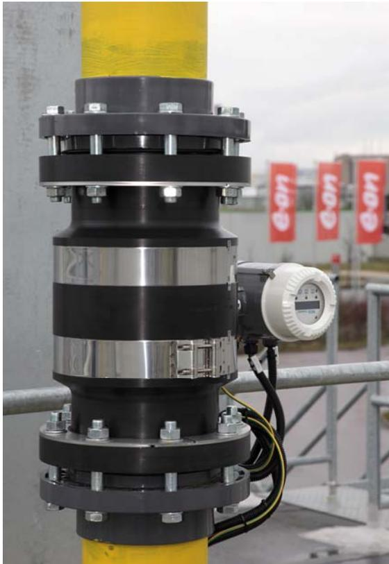
Figure 7: Installation of an ultrasonic gas meter in the Schwandorf plant
