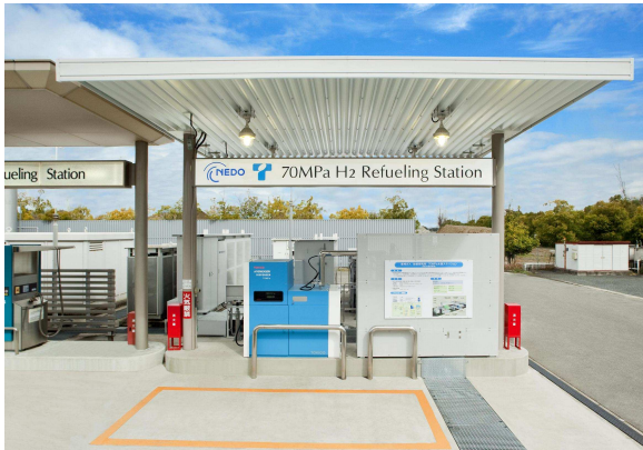
Photo.2 Appearance of the 70 MPa hydrogen refueling station in Toho Gas Technical Research Institute
