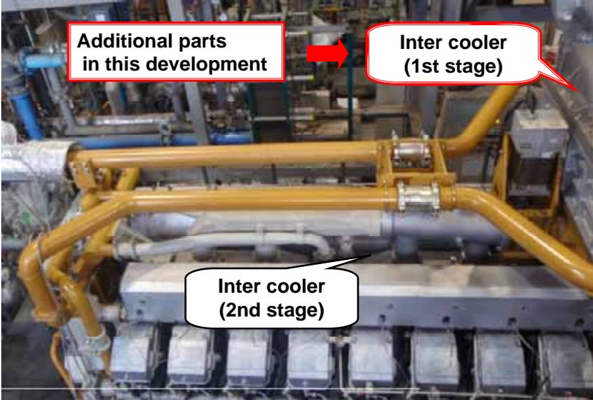
Figure 12 The development of new heat recovery system (2-stage inter cooler)
