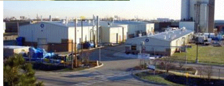
Energy & Environmental Technology Center
