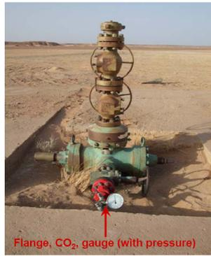
CO<sub>2</sub> breakthrough occurred at KB- between inspection intervals (August 2006 to June 2007)
