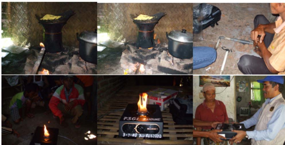
Figure 5. Visit to a house at south of Indramayu City – West Java Province. The residence has used biogenic gas as their energy source for daily cooking. A simple technology has been applied by the residence; the gas is piped through PVC tube from the source – a hand auger well, to an iron tube in the kitchen. The figure shows that the iron tube was replaced by a specially design low pressure stove donated by MGI.
