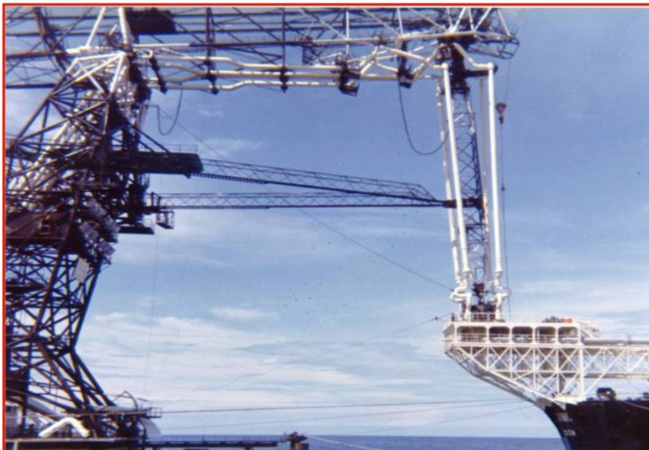
Figure 2: Shell Brunei LNG Crane loading system with stern loading. Exposed location.
