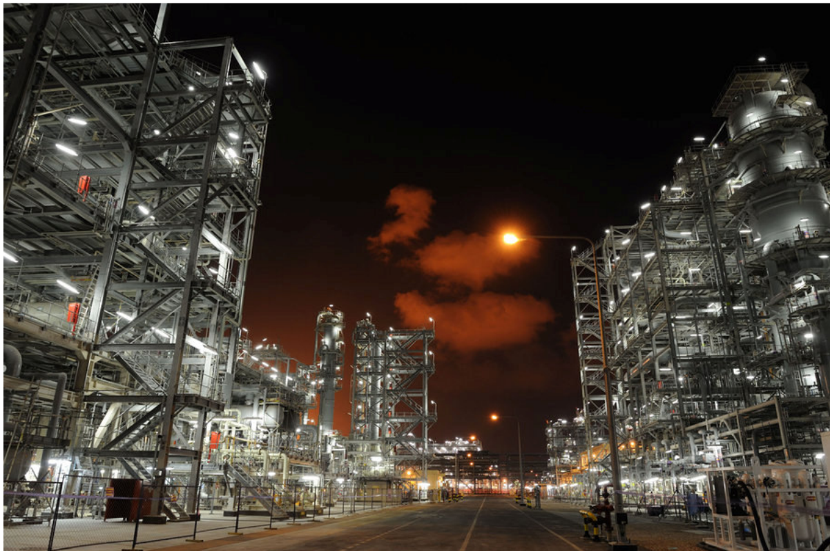
Image 2 – Pearl GTL liquid processing unit
